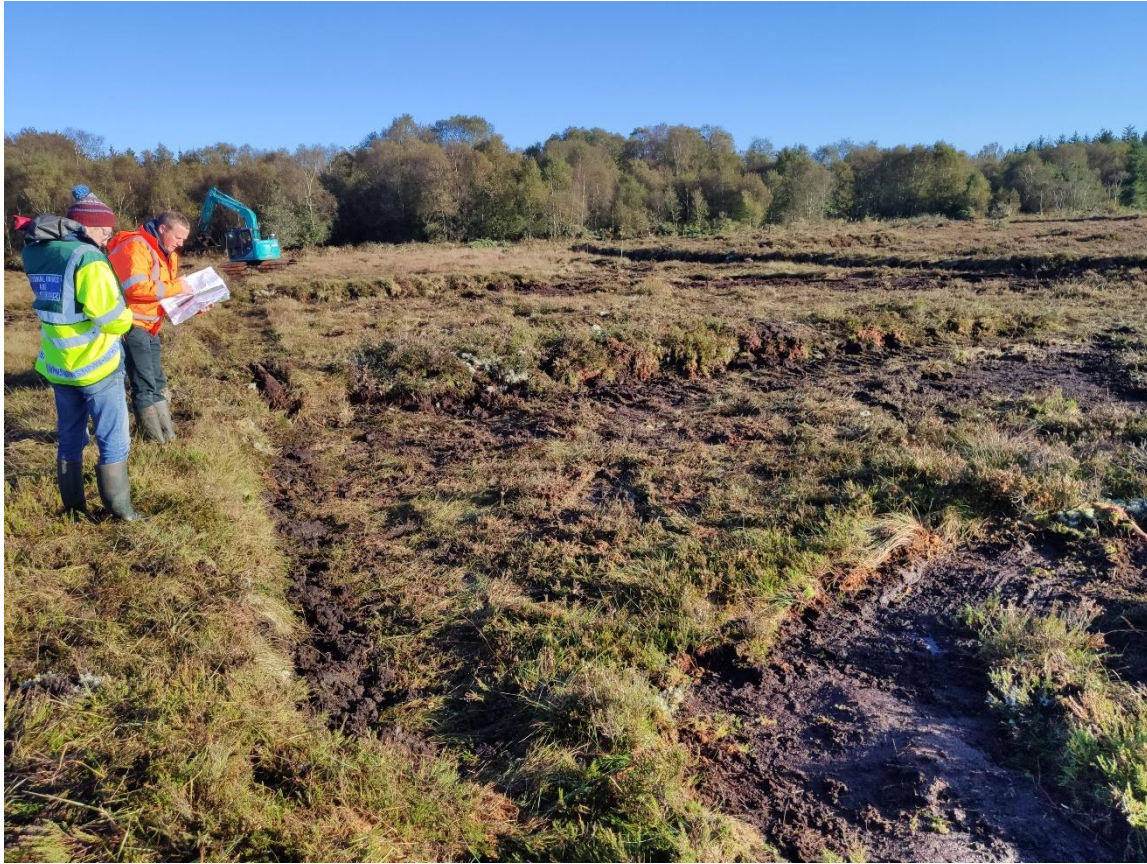
Starting cell bunding Cloncrow Bog NHA
